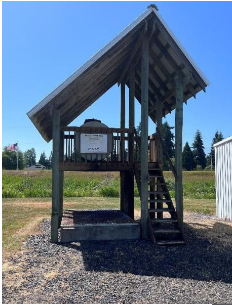
Figure 1-16: CLS Oil Recycling
