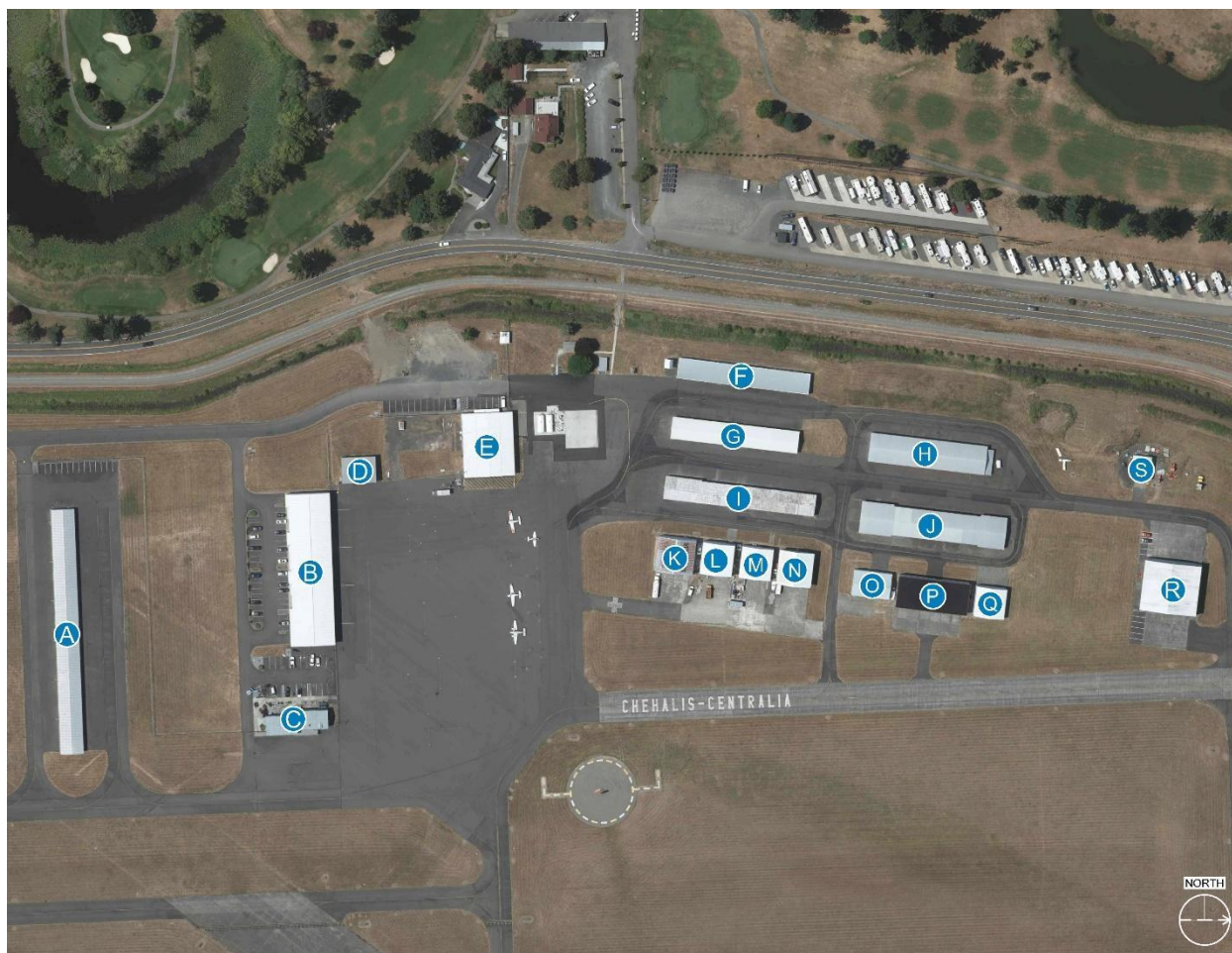
Figure 1-13: Hangar Locations at CLS
